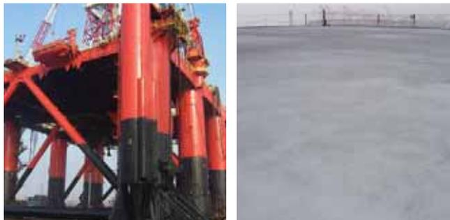
The rig 'Nan Hai 2', owned by CNOOC, during application of Jota Armour. A 200 µm coat of Primastic Universal was applied to the zinc silicate shopprimer (20 µm) followed by an 1800 µm coat of Jota Armour Grey. After touch up a 60 µm coat of Hardtop AS Green was applied.
