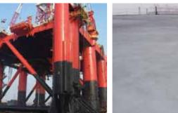
The rig 'Nan Hai 2', owned by CNOOC, during application of Jota Armour. A 200  $\mu$ m coat of Primastic Universal was applied to the zinc silicate shopprimer (20  $\mu$ m) followed by an 1800  $\mu$ m coat of Jota Armour Grey. After touch up a 60  $\mu$ m coat of Hardtop AS Green was applied.
